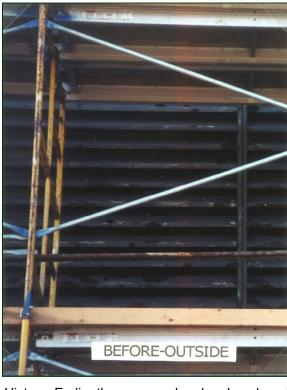
Challenge: Both sides of an air inlet grill (1,200 square feet of surface area) were covered with aging Lead-Based Paint (LBP) in damaged condition that was damaged. Also, visible evidence of mold and mildew and metal corrosion existed in a few spots. For air quality and visual appearance reasons, the owner of this major Midwest headquarters site wanted a quick and affordable solution.
