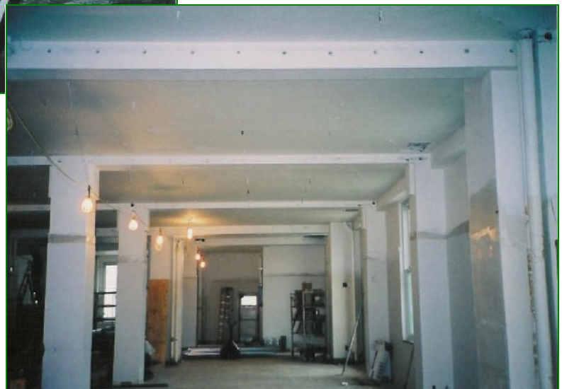
Ceiling of Room After Encasement
