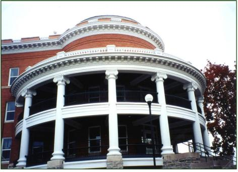
Challenge: Badly deteriorated Lead-Based Paint (LBP) on metal and wood ornate trim at the Minneapolis Veterans Home would have required extensive time and expense to remove by any of the means usually employed for removal, such as scraping or the use of chemical strippers. Removal of the damaged paint also posed a real risk of damage to the ornate surfaces of this historic structure.
